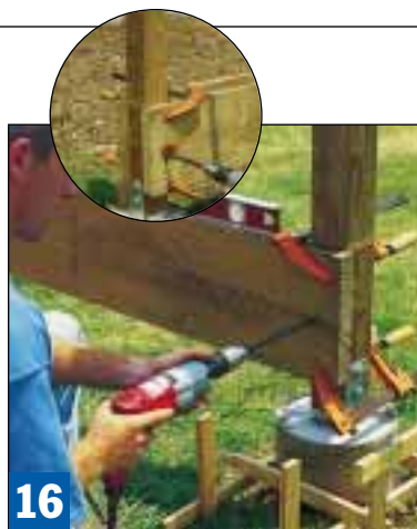
16 When the beams go up, clamps hold them until you get height and level adjustments made. Then drill and bolt.
