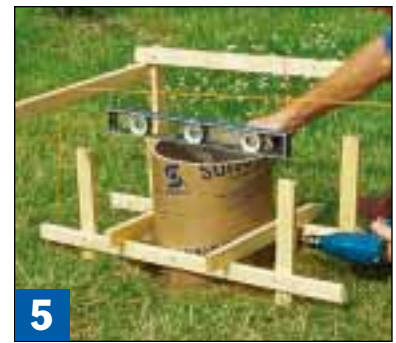
5 Rest a second pair of crossbars on the first pair, check the form for level in the other direction, then drive screws to “lock” the form where it sits.
