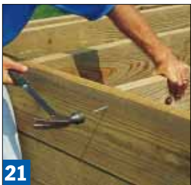
21 After bolting the rim joist to the posts, nail through it into the end of each joist. Check joist alignment as you go.
