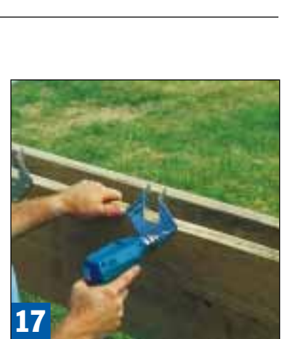
17 Transfer the joist layout marks from the ledger to the beam, then fasten a hurricane tie at each joist location.
