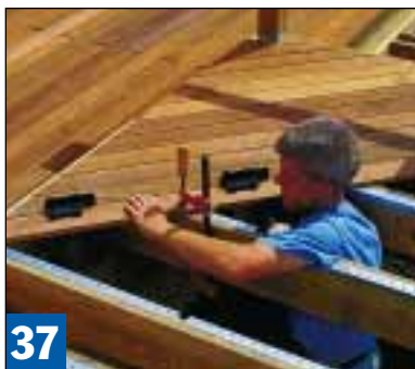
Orienting decking diagonally defines height changes between levels. Use clamps to keep boards from shifting.
