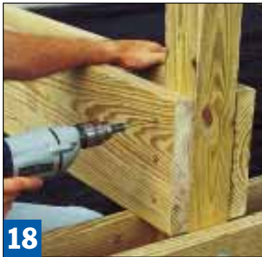
18 Install the joists at each post first, with the ends flush with the post face. I used Simpson 'SDS' lag screws here.
