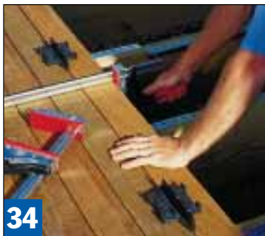
Clamps can coax crooked boards into a straight line before you fasten them. Always use spacers for a uniform gap.
