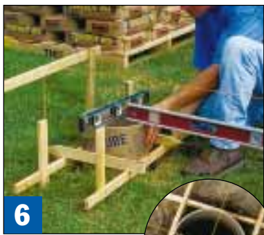
6 Keeping the forms level to each other looks best, but sloped terrain might require multiple levels.
