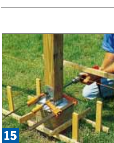
15 With the post base still clamped, drill through the bolt holes in the metal bracket and install the bolts and nuts.
