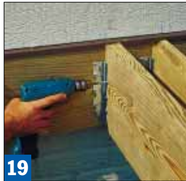
19 Use screws to secure the joists in their hanger brackets, and fasten at each hole for maximum holding power.
