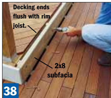
The diagonal decking orientation will require an extra 2x8 subfascia (with 1/2" spacers) to support the ribbons.
